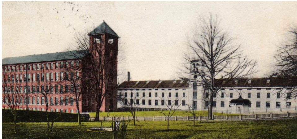
The New England Mill buildings. The brick factory still stands near the intersection of Vernon Avenue and Brooklyn Street.
